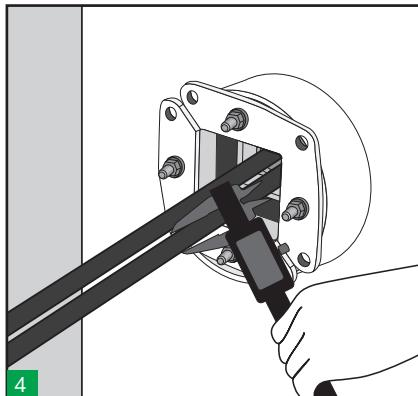
4 Take measures of the cables diameters and select the appropriate HTS Tolerant blocks. Colour code will help you to select the correct ones.
