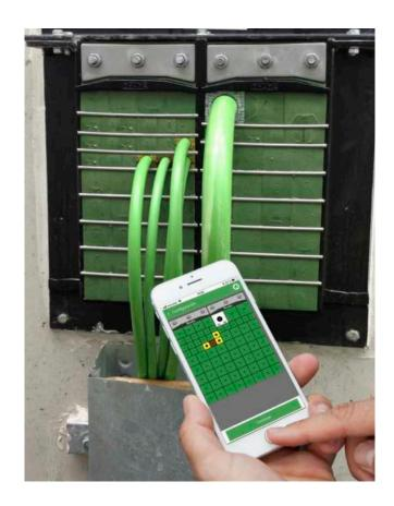
Designed to be launched from a portable device iOS or Android (smartphone or tablet). The Installer's App allows the installer to calculate automatically the best configuration for a transit, it exports the material list, drawings with colourcoding and other important information.
